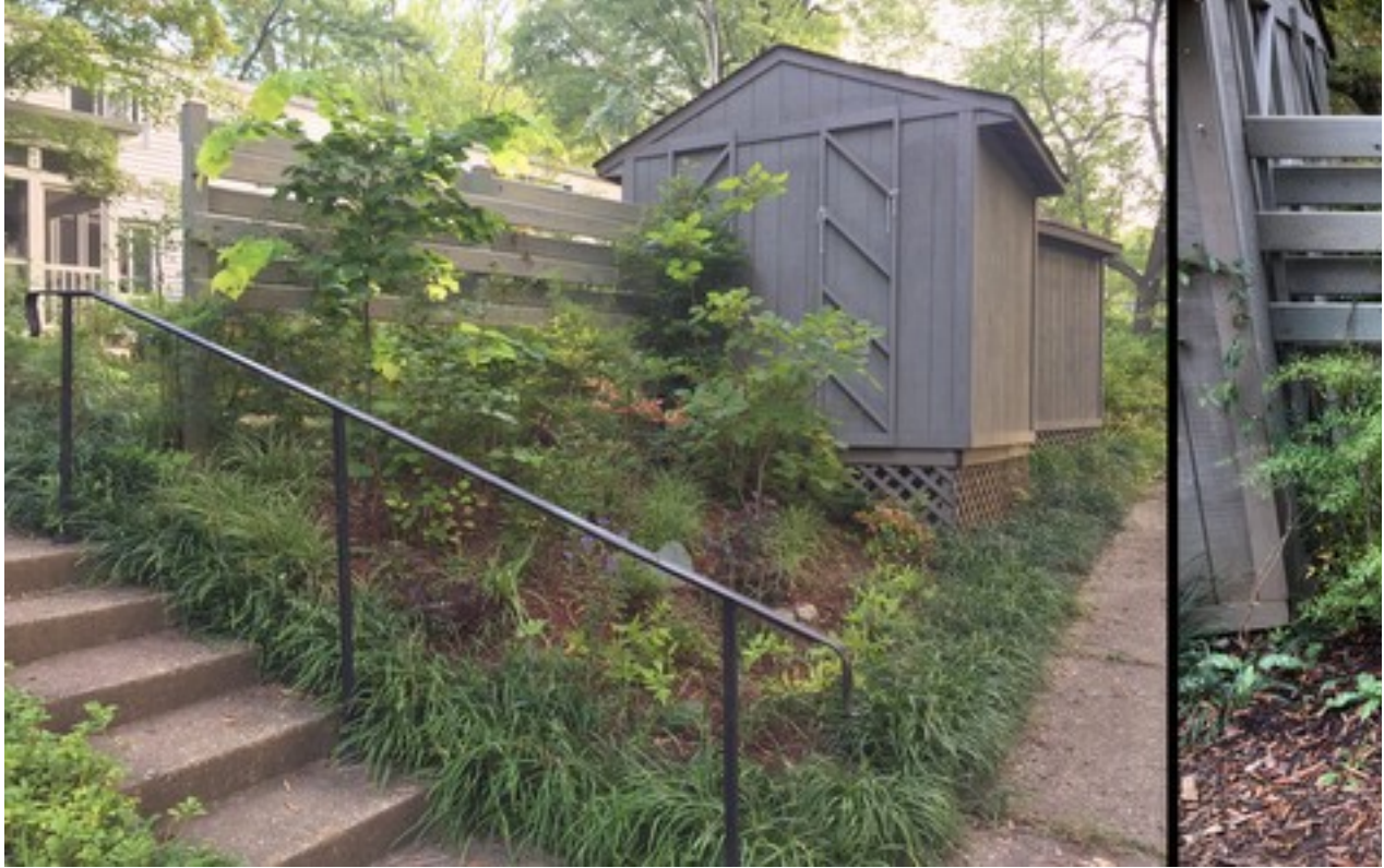
Example of targeted and limited screening in a GHI yard: only 3 feet tall, mounted 3 feet above ground level, about 12 feet away from the sidewalk.
