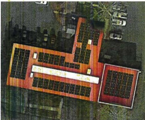
Admin Building Roof Mount
