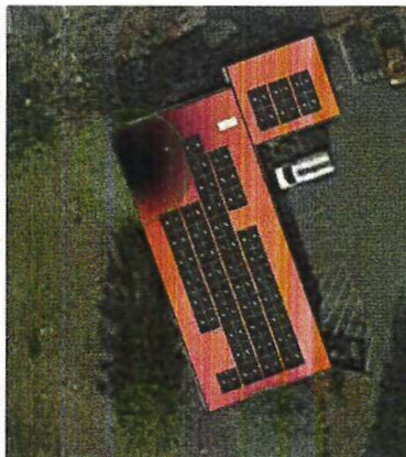
Warehouse Building Roof Mount
