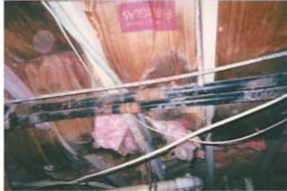
Fiberglass installed upside down
