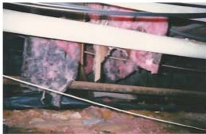
Fiberglass Batts Falling Down
