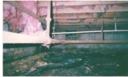
Vapor barrier not extending to wall
