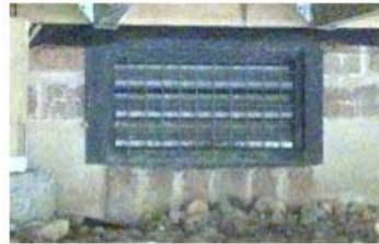
Auto vent (GHI's final fix after animal intrusion in late 2007). Vent below permanently mounted by member contractor in 2014
