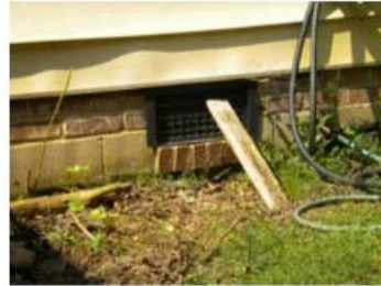
Auto vent (GHI's final fix after animal intrusion in late 2007). Vent below permanently mounted by member contractor in 2014
