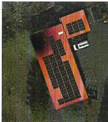
Warehouse Building Roof Mount
