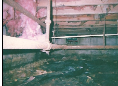
Actual GHI crawl space (before upgrades)
