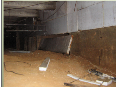
Before crawl space upgrades
