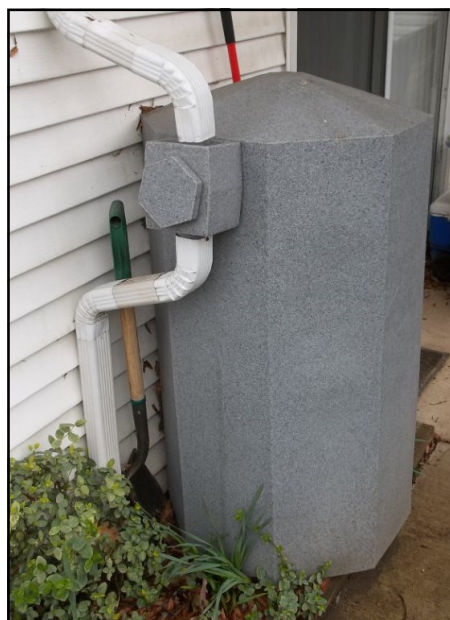
Installed rain barrel. GHI photo.
