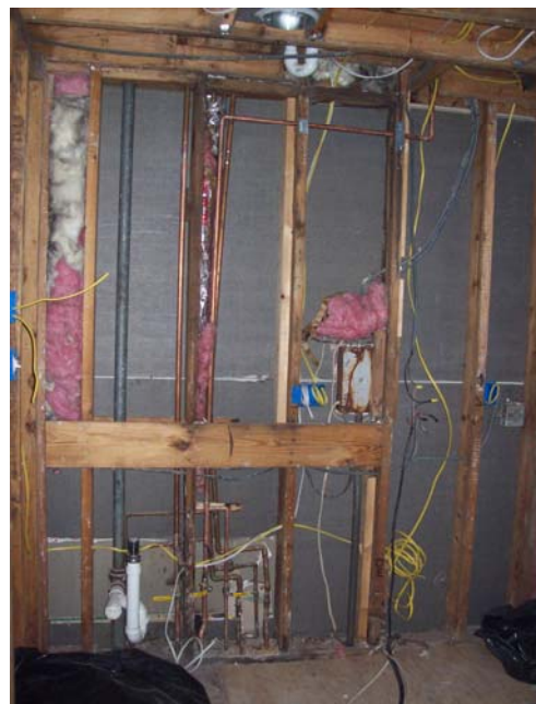
Interior wall during a renovation Photo Credit: Tom Sporney
