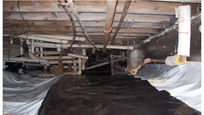
Frame crawlspace after improvements. Photo by GHI.
